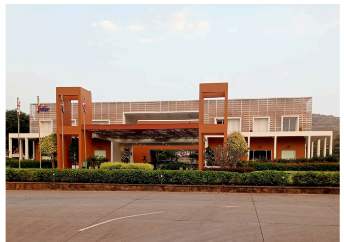
Image 1: Inspire Institute of Sports Building and infrastructure
