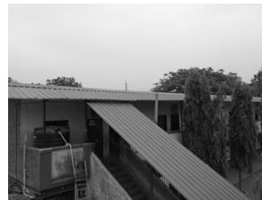
Replaced roofs with safe and durable roof panels
